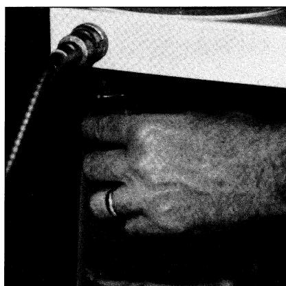
4. Drop pump body through mounting hole so that switch faces right side of tank. Slip plastic tube connected to pump discharge into hole nipple.
